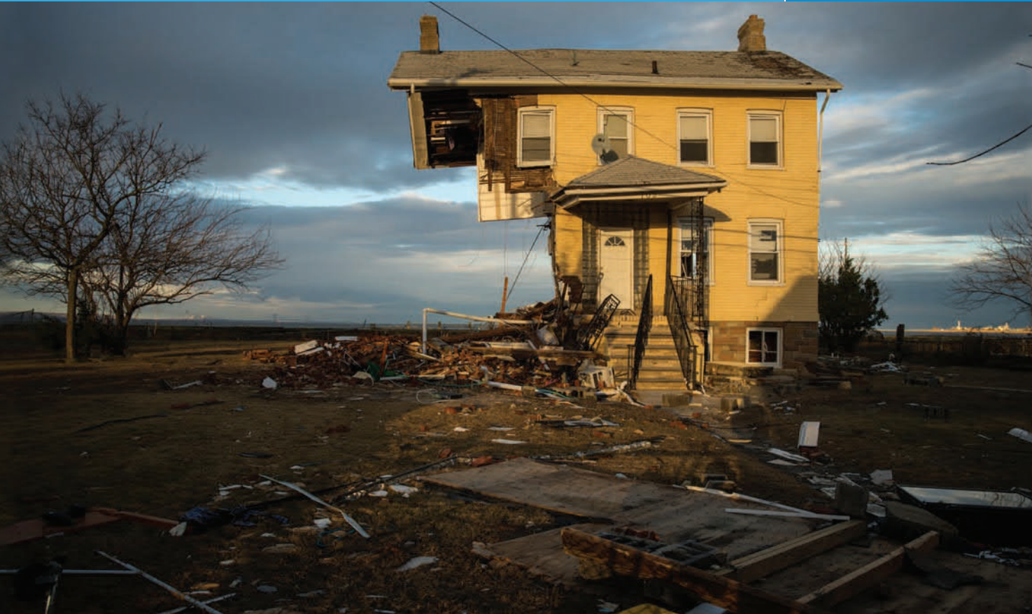
A destroyed home in Union Beach, New Jersey, following Hurricane Sandy hitting the coast of New Jersey and New York in November 2012.
